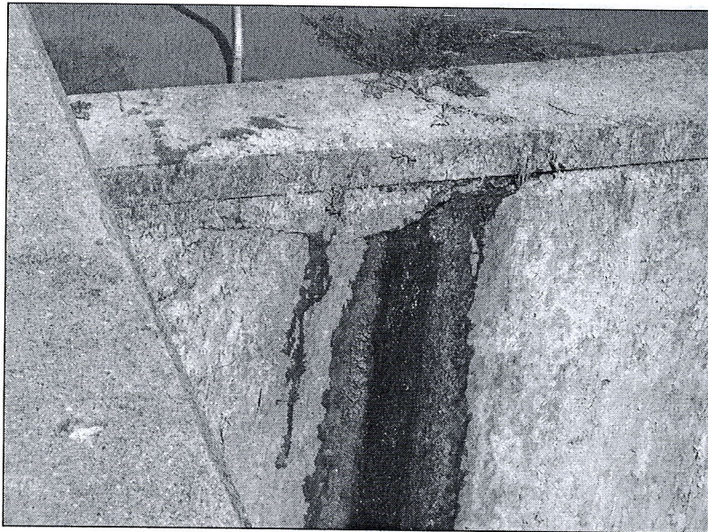
Leak at fixed crest
