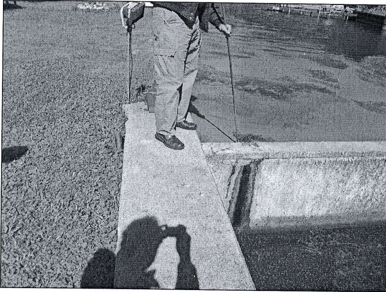
Leak at fixed crest
